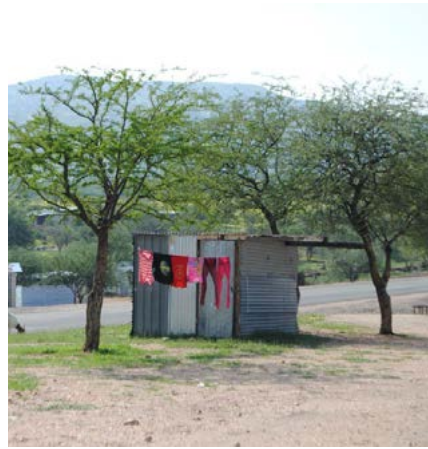
Image 8-9. An 'informal' structure in Namibia.
