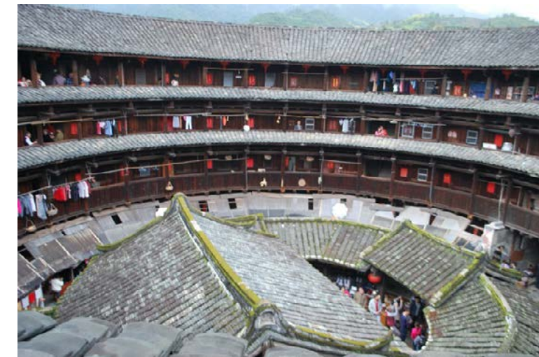
Image 8-10. Communal housing in traditional rammed earth Tulou, Fujian, China
