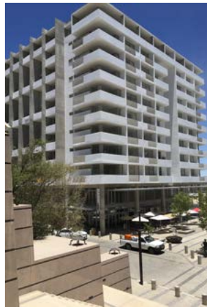
Image 8-8. Freedom Plaza apartment building in Windhoek, Namibia. 6
