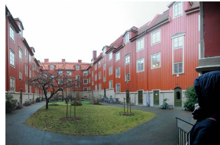
Image 8-13. 18 th -Century working class housing, now gentrified; Gothenburg, Sweden.
